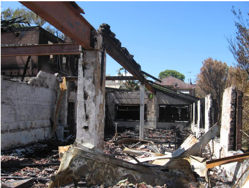
Figure 3 — north-east view along the former dining room (Rooms 14 and 15) revealing the steel beams from a phase of alteration.
