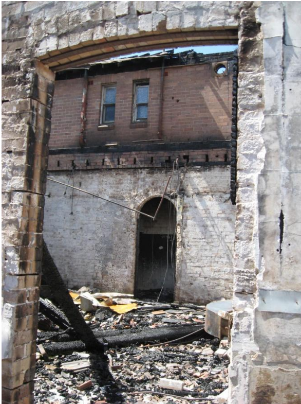
Figure 4 — north-east view across the original locker room (Room 16). This was one of the most intact rooms with timber panelling.
