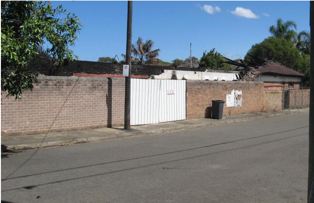
Figure 2 — southwards view from Bowlers Avenue showing destroyed roof.
